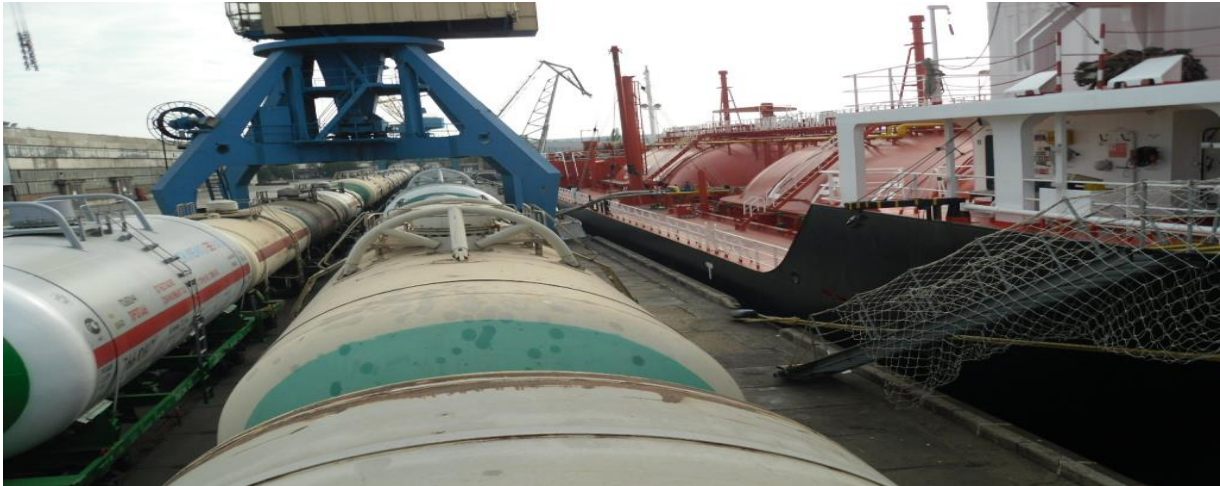
Figure 3. Unsafe Ship-Shore Access
